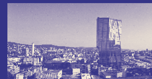
03 Prime Tower | Gigon Guyer Architekten
