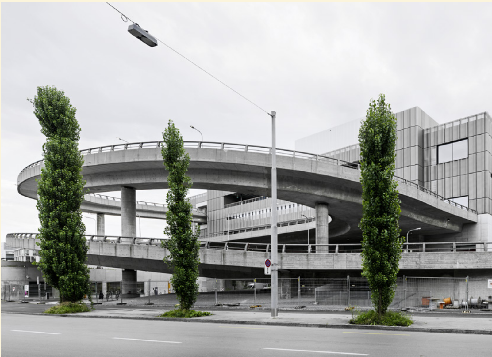
↑ Winding its way past five floors is a concrete ramp that now serves as the building's vertical boulevard. Photo Simon Menges
